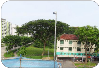
Figure 3: Bullet camera mounted on a specially erected support at a site under construction
