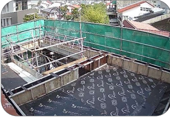
Figure 6: At a floor of a building under construction
