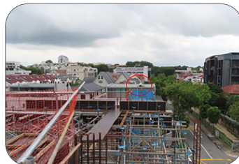
Figure 5: Construction of support structure
